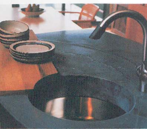
A concrete countertop, LEFT, can be paired with a wood cutting board. Concrete fabricators can create a multitude of colors, BELOW, by adding powdered and liquid pigments.
