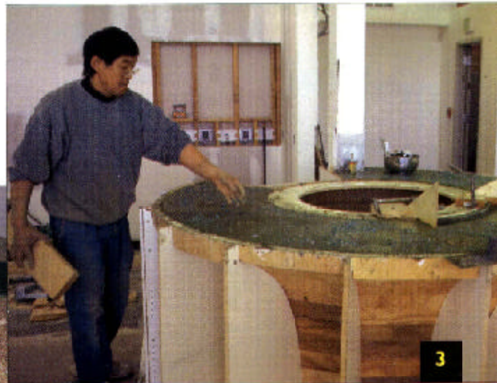
(Top) Plywood formwork with cast plaster mold; (middle) central column of formwork in place before pour; (bottom above) Fu-Tung Cheng overseeing concrete pour; and photographs of completed counter.
