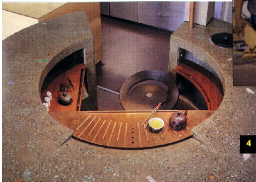
(Top) Plywood formwork with cast plaster mold; (middle) central column of formwork in place before pour; (bottom above) Fu-Tung Cheng overseeing concrete pour; and photographs of completed counter.
