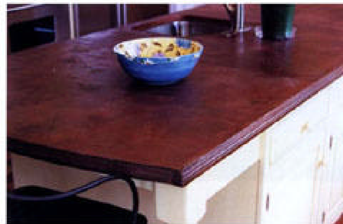
Concrete can be dyed, shaped and installed in a thick slab for a massive look. Courtesy The King's Grant
