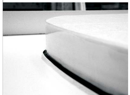
Image 3: Sealing the base
