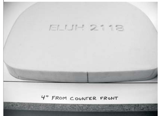
Image 2: Placing the form
